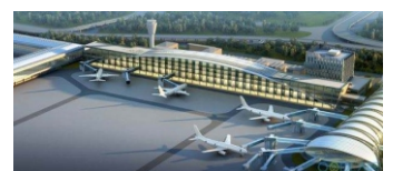
▲机场应急供电 Emergency Power Supply At The Airport
